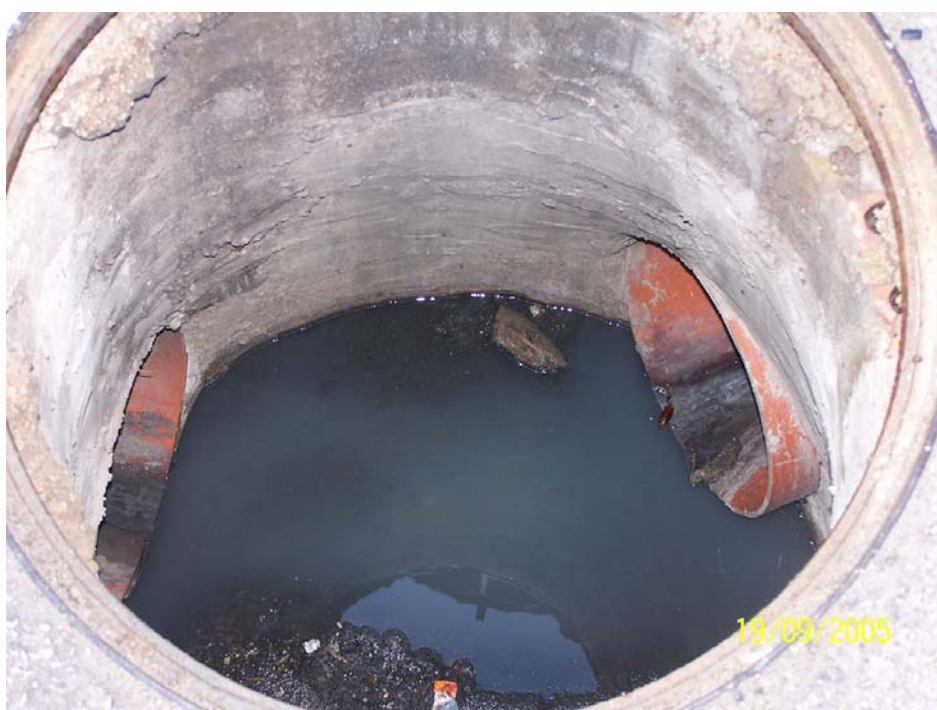
Interior del colector
